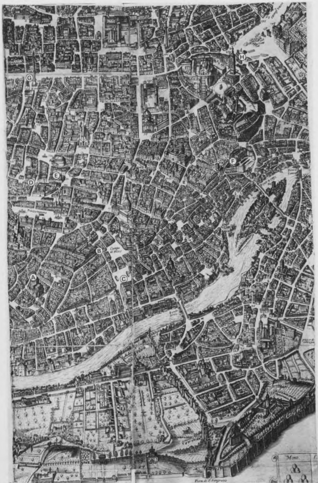
Text ill. 3. A: Church of Sta Maria in Vallicella; B: The Cancellaria (the Palace of Cardinal Montalto); C: Farnese Palace; D: Church of S. Luigi dei Francesi; E: Giustiniani Palace; F: Savelli Palace, formerly the Theatre of Marcellus; G: Column of Trajan; H: Temple of Vespasian
